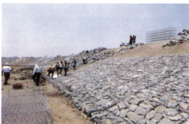
Stone pitching for slope protection work in progress, Odisha. Saline Embankment at Keutanjanga, Odisha.
