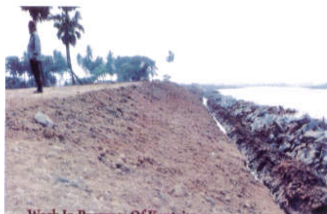
Stone pitching for slope protection work in progress, Odisha. Saline Embankment at Keutanjanga, Odisha.
