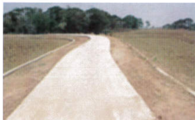
Cement Concrete (CC) Road at Nachhipur, Bhadrak District, Odisha
