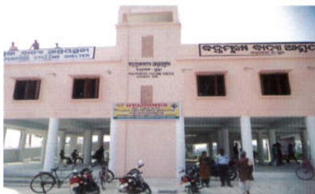
Multi Purpose Cyclone Shelter at Bajrakota, Odisha
